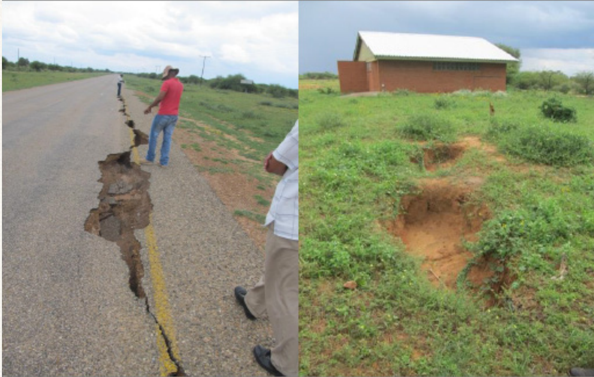
Figure 11: a) A Damaged road in Hatsalatladi due to fissuring; b) Earth fissures within Hatsalatladi primary school premises.
