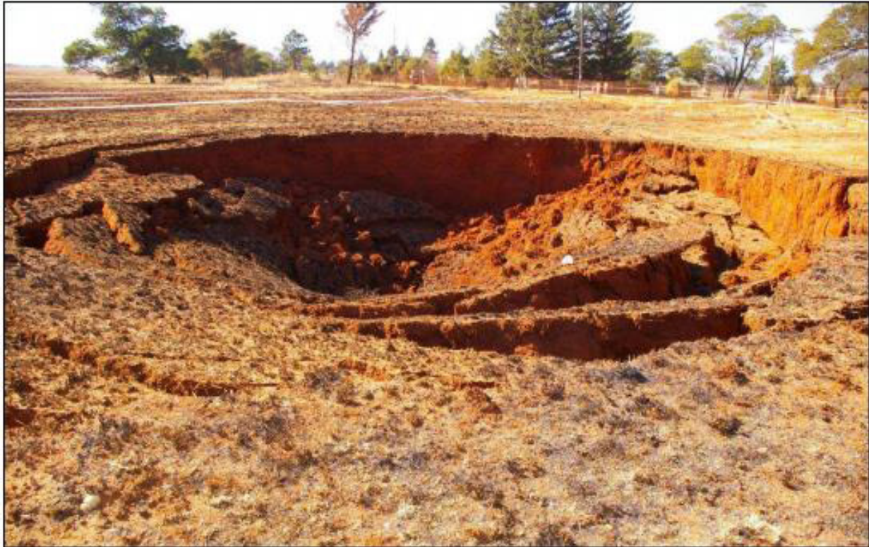
Figure 5: Typical Dewatering subsidence (CSGS 2011).
