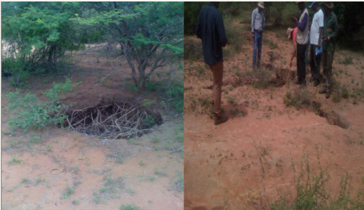
Figure 12: a) a depression observed in affected area; b) tripple junction of different trends of earth fissures in Ditshukudu, Kweneng District.
