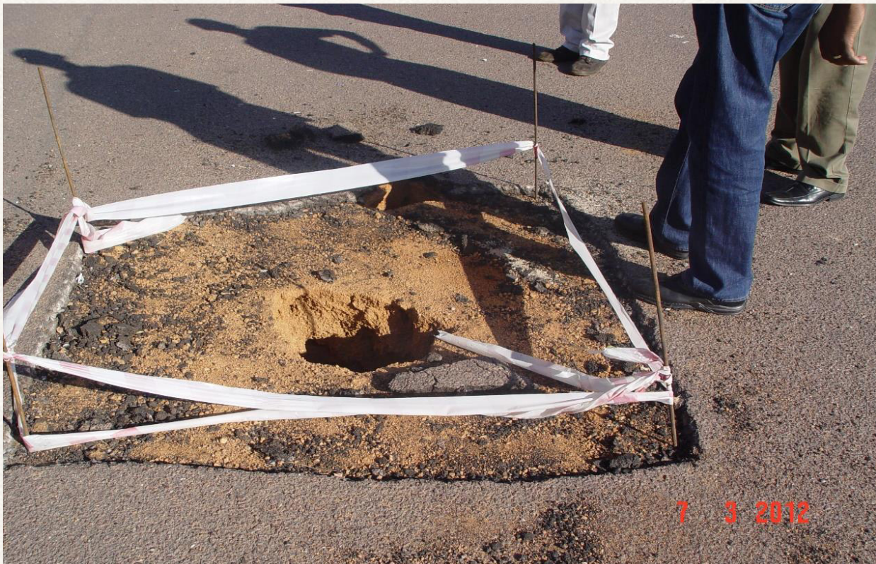
Figure 13: A sinkhole that occurred in Lobatse, South East District.
