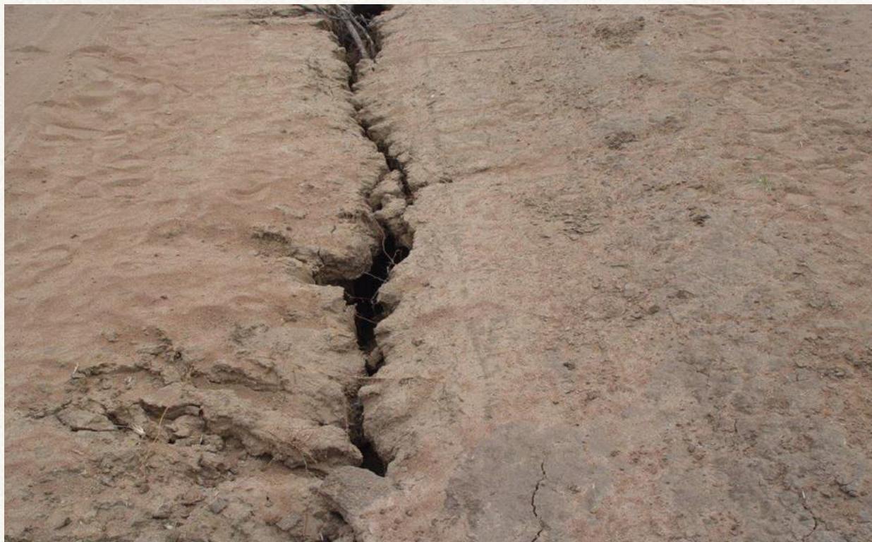
Figure 9: Earth fissure in Makapane
