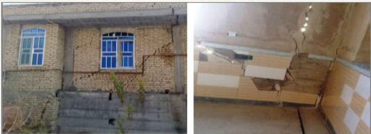
Figure 7: Diagonal, Tapering cracks, typical sign of subsidence on buildings (Hossein Rahnema, Sohrab Mirasi, 2012).
