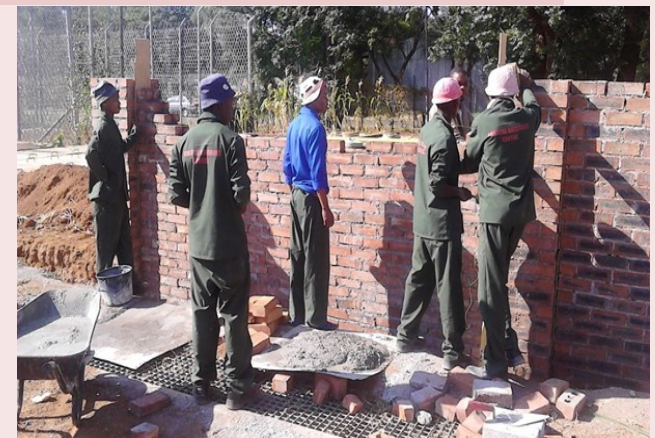
Construction of a brick wall using Manufactured sand as a mortar
