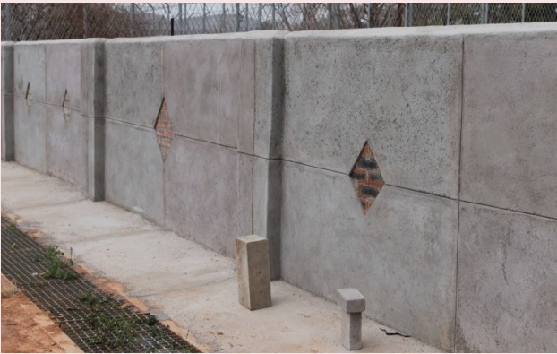
Experimental wall at Geological Survey in Lobatse, the wall is built from different brick types and plastered using sieved and un-sieved manufactured sand.
