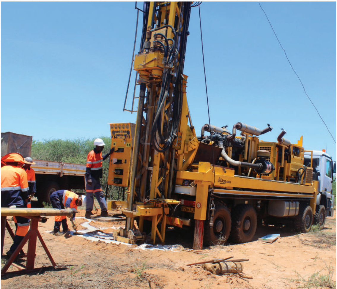
Picture: Drilling - Cement grade and calcrete deposit (Letlhakane)
