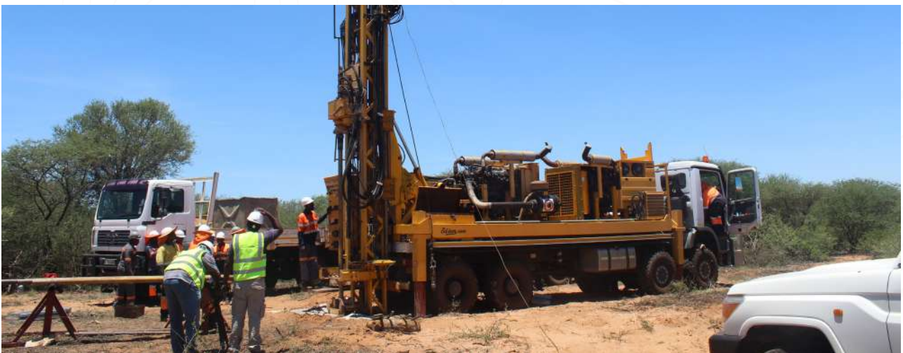
Figure 20: Borehole drilling
